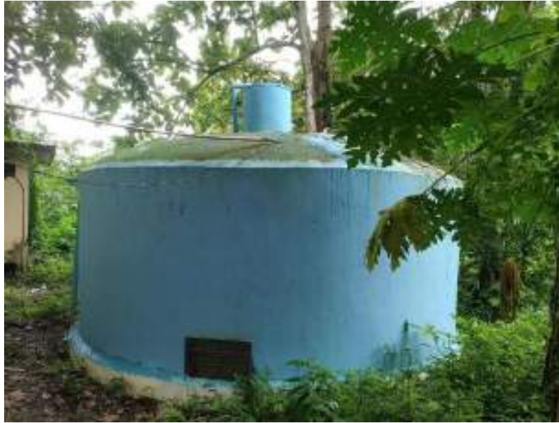
Figure 11 RAIN WATER COLLECTION STORAGE
